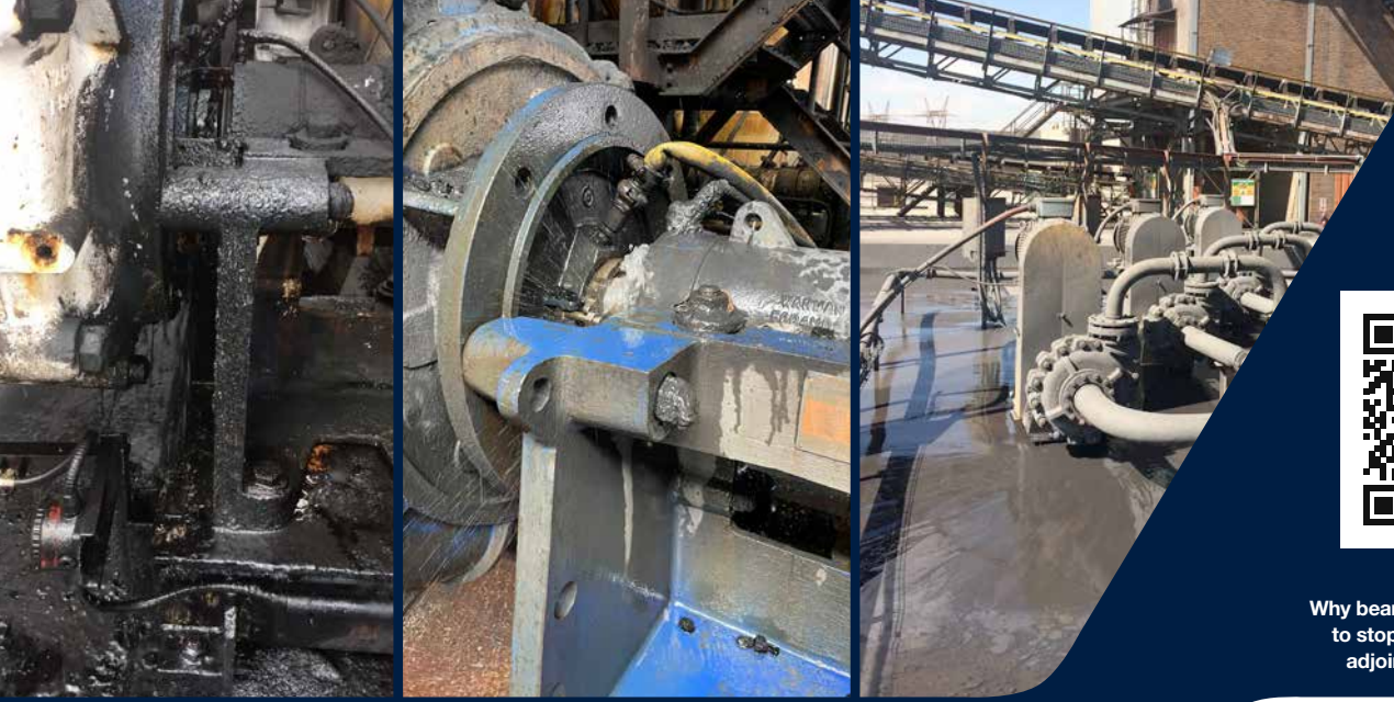
Slurry Leakage
