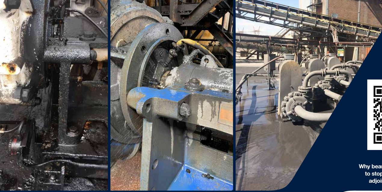
Slurry Leakage
