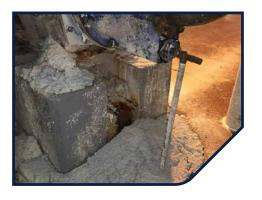
Arjowiggins asked AESSEAL to install a new sealing system on one of the refiners to test its efficacy. AESSEAL replaced the traditional packing with CDSA double cartridge mechanical seals and a SWFF-TF seal support system.
