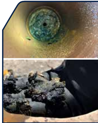
Before - solids inside vessels
