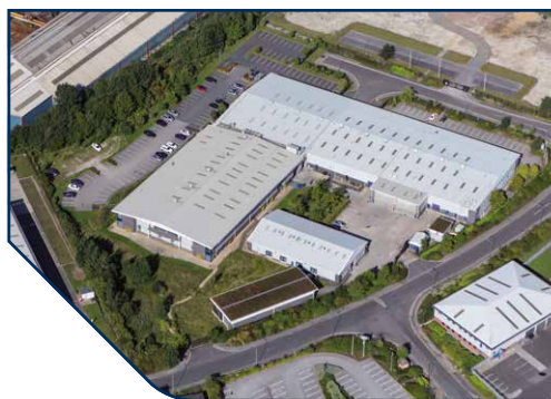
AESSEAL Centre Technologique International
