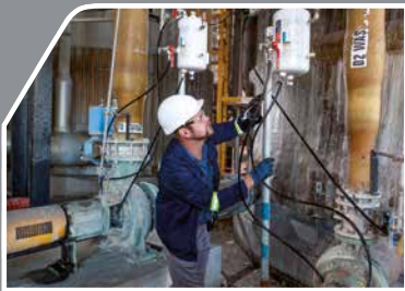
Engineer installing continuous loop system
