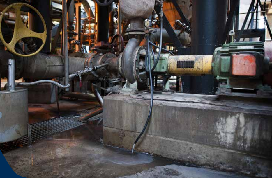
(left) Before the AESSEAL® solution: Pump and mechanical seal, fitted with quench-to-drain flushing system.
