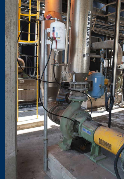
(left) Before the AESSEAL® solution: Pump and mechanical seal, fitted with quench-to-drain flushing system.
