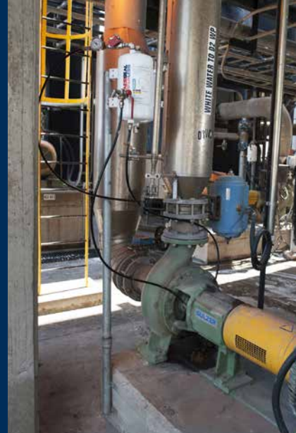
(left) Before the AESSEAL® solution: Pump and mechanical seal, fitted with quench-to-drain flushing system.
