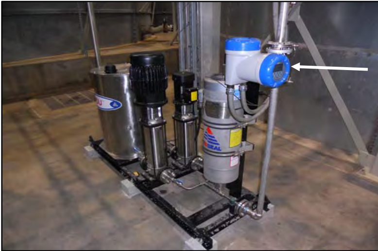
Figure 18. Skid-mounted FDU unit with digital flow meter (arrow) provides pressurized water for seal barrier fluid.
