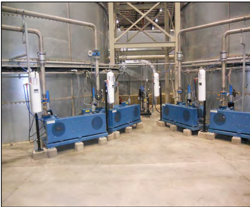
Figure 16. Four of the 16 Warman pumps serviced by the pressurization skid in the background.
