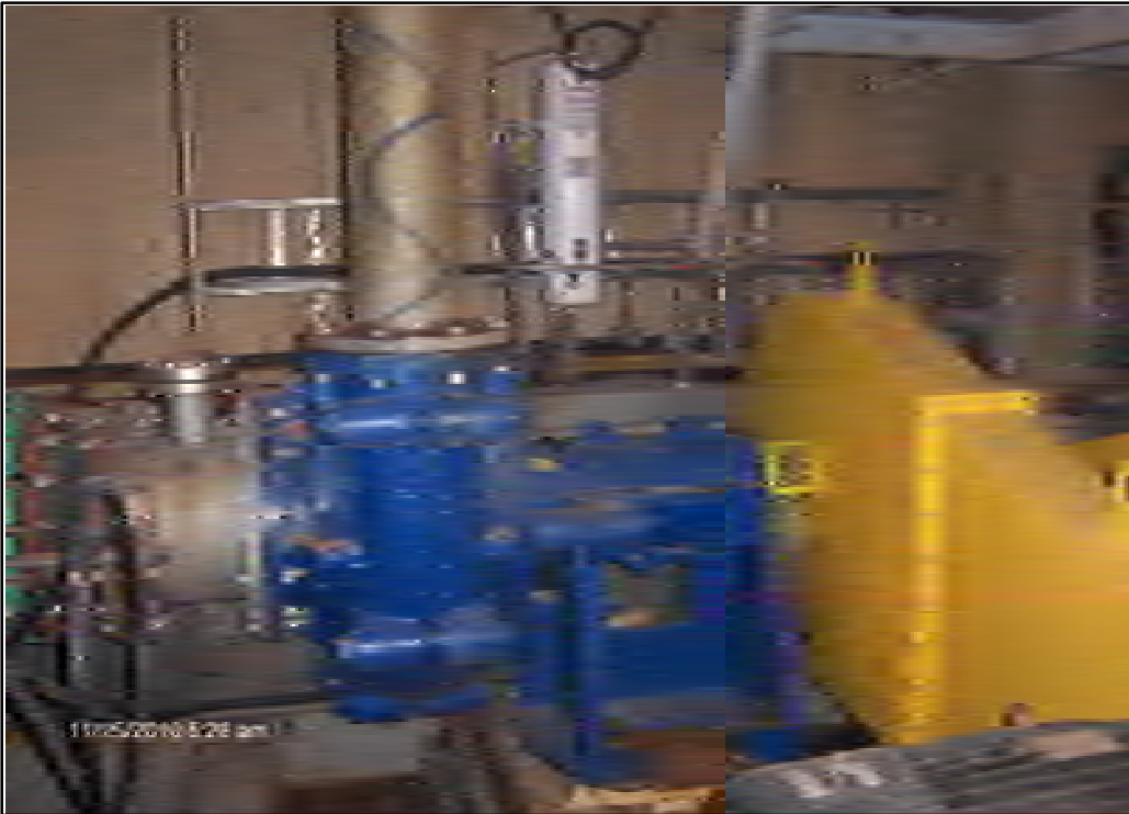
Figure 13. Warman AH-F Froth feed pump, fitted with double mechanical seal and tank system.
