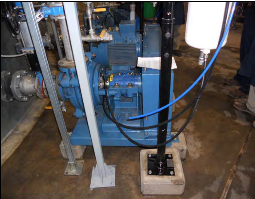
Figure 15. Warman slurry pump showing double mechanical seal and white tank.
